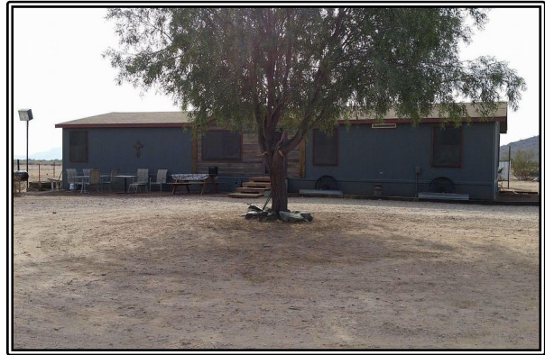
1309 South 393 rd Avenue
