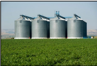
Grain Storage Facility
