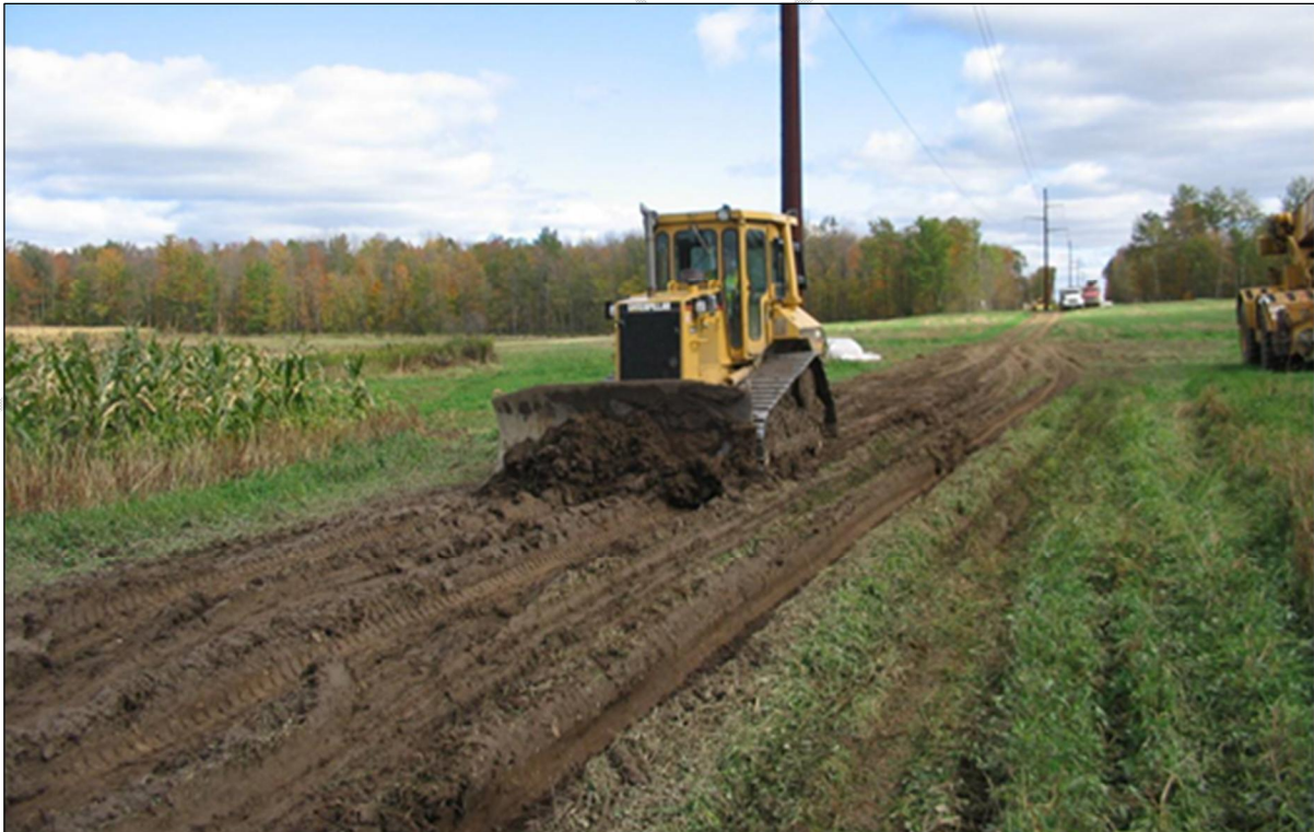
Figure 5-2 Ruts being smoothed with blade. Soil is not waterlogged as shown in Figure 5-1.
