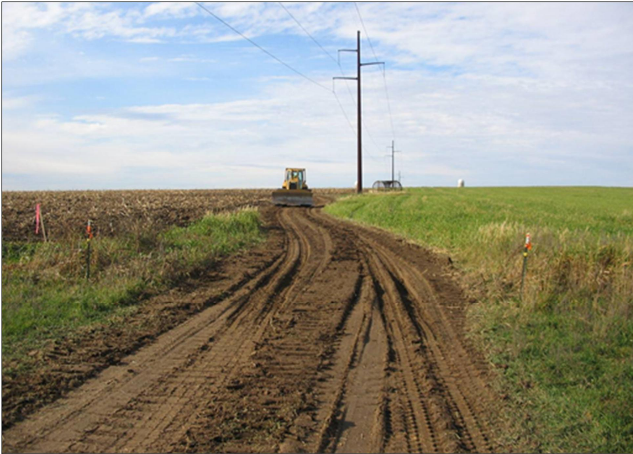
Figure 5-3 Smoothing out ruts by backblading with a dozer
