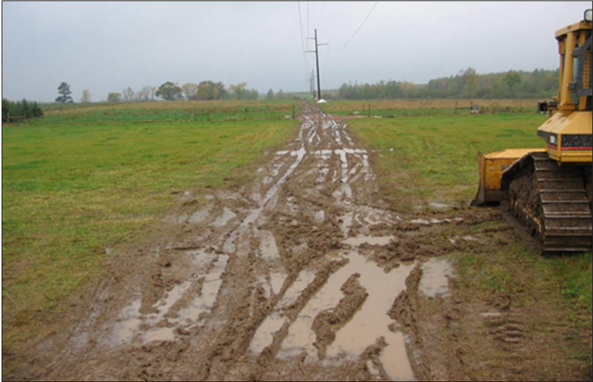
Figure 5-2 Ruts being smoothed with blade. Soil is not waterlogged as shown in Figure 5-1.
