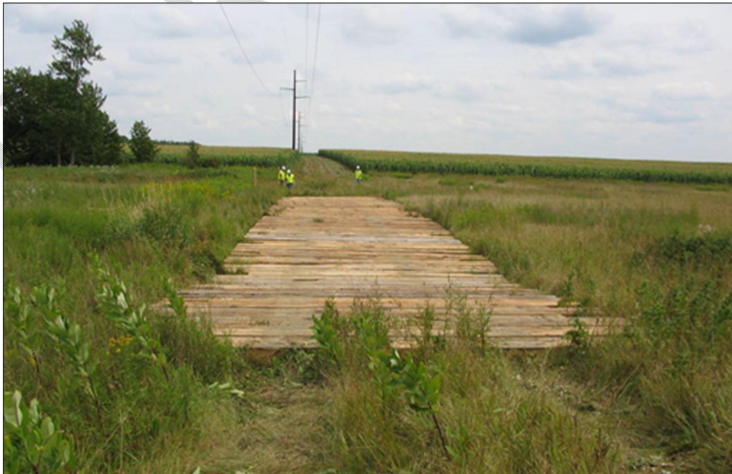
Figure 5-4 Timber construction mats in a wet meadow wetland
