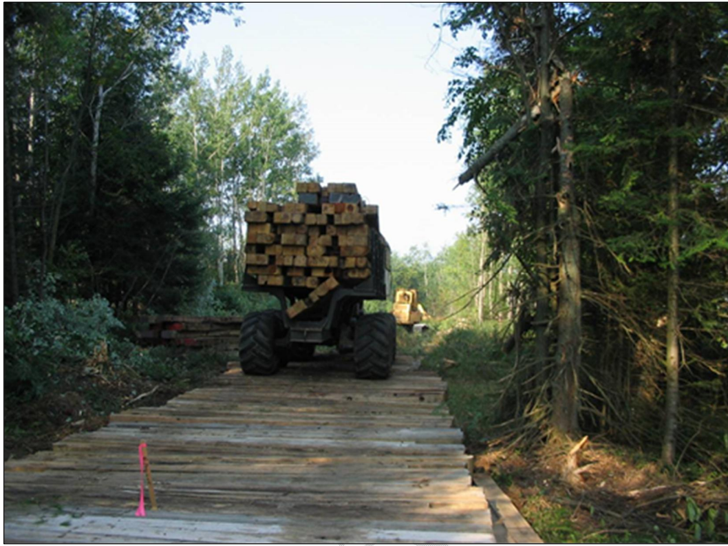
Figure 5-5 Timber mats being placed in a forested wetland. Tracked vehicles and high flotation tires can be used in some instances in lieu of mats.
