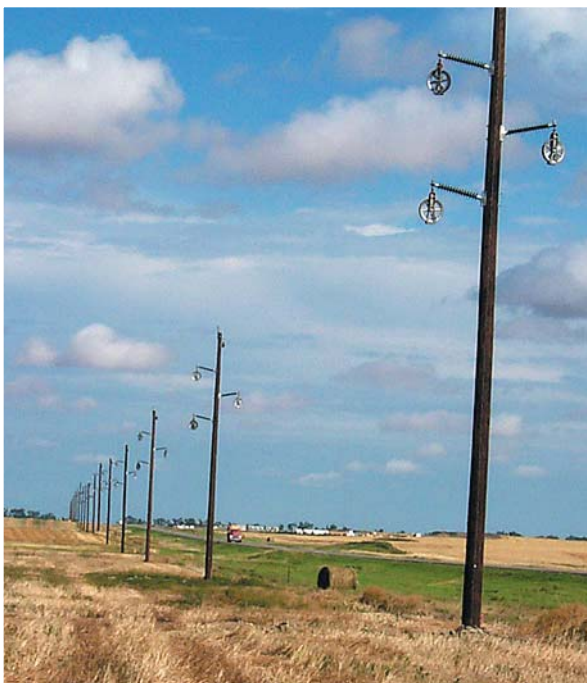
Pulleys are attached to transmission poles to string lines. (Photo by Ron Beneda, Cavalier County Extension Agent)
